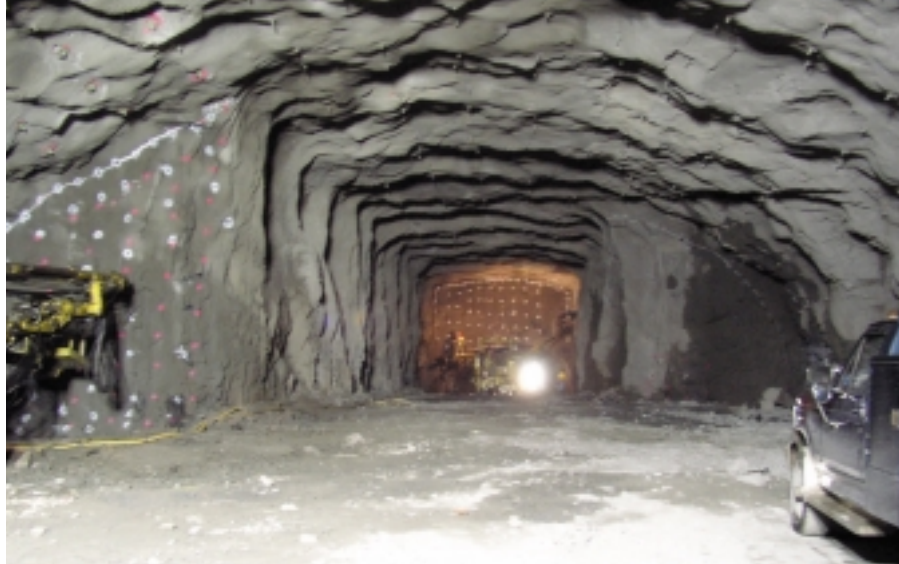
Centre heading and station slash rounds being drilled
