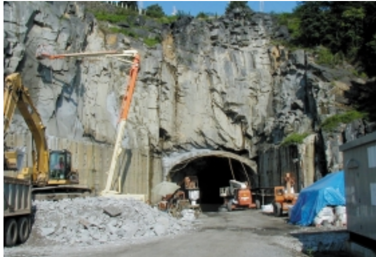
Weehawken tunnel east portal
