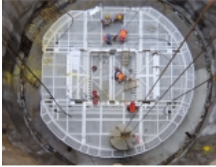
Work deck stage in shaft
