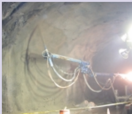
Meyco shotcrete robot in use at the Weehawken tunnel
